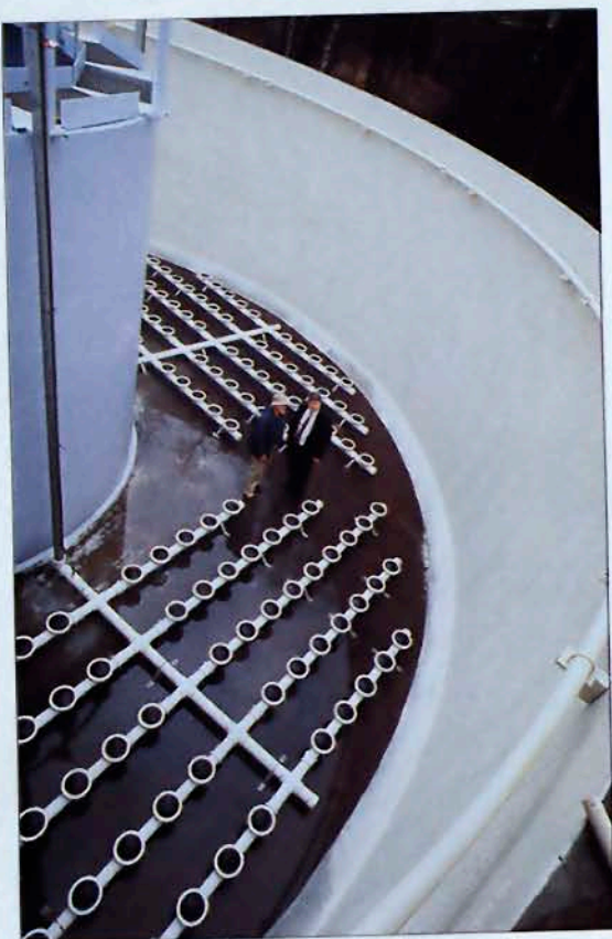
Course bubble diffusers were replaced with PVC piping and fine bubble diffusers to enhance aerator biological decomposition efficiency.
