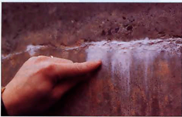
Sulfuric acid and hydrogen sulfide generated by the sewage treatment process caused extensive corrosion, including damage to the concrete walls evident in calcium staining on the exterior of the clarifiers.
