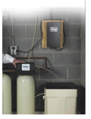
but usually the problem is a fouled mineral bed. Check the backwash, brine draw and brine tank fill times. Then increase the frequency of regeneration.
