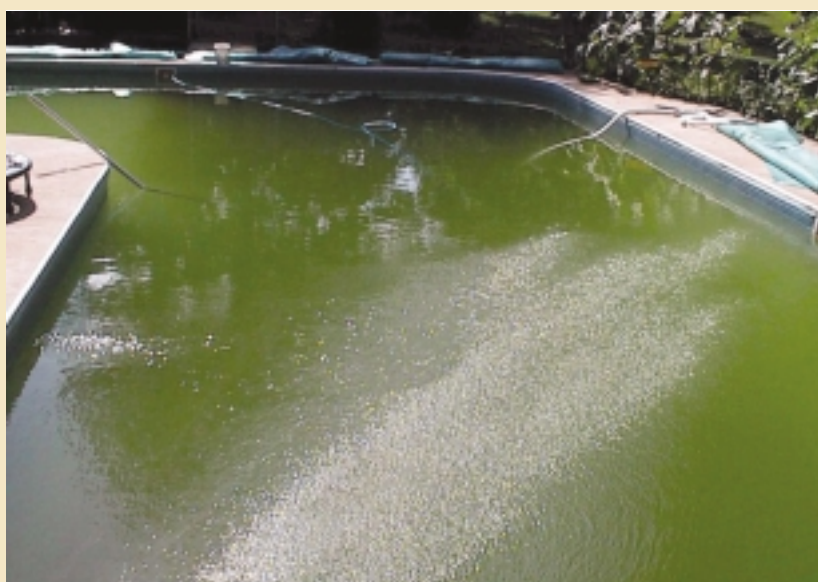
Picture A. Just a few weeks after an ionization, ozone and chlorine injection system was installed. Iron is removed from the pipes and causes the brownish-green color.
