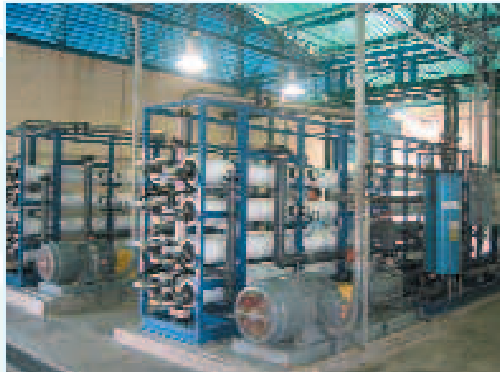
ITT -Aquious reverse osmosis desalination system pumps 1.5 million liters of water per day to Taos residents.
