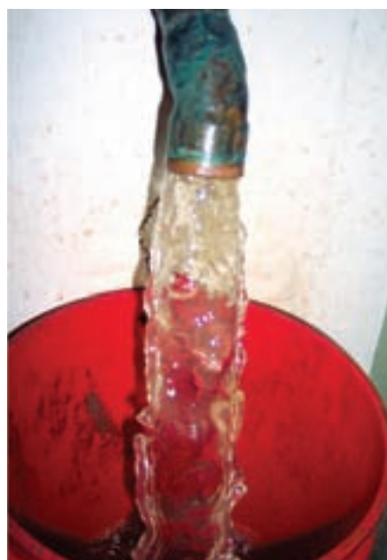
Because of the amount of iron present, the unit needed to be flushed with acid. Aqua Ion Plus+ backwashed both tanks until the water was clear.
