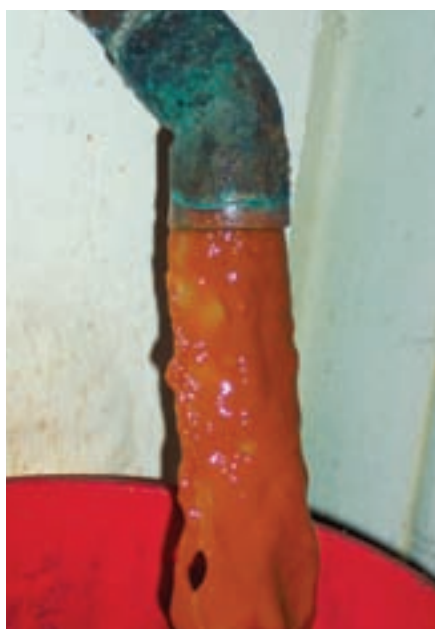
Because of the amount of iron present, the unit needed to be flushed with acid. Aqua Ion Plus+ backwashed both tanks until the water was clear.
