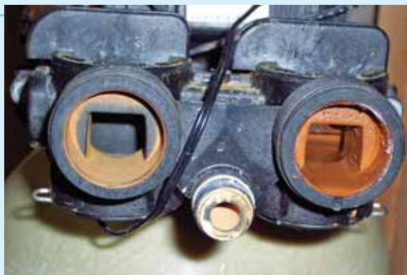
Top Left: Example of proper configuration of an iron filter with BIRM on right and a softener with a mixed bed of cation and anion exchange media on left.
