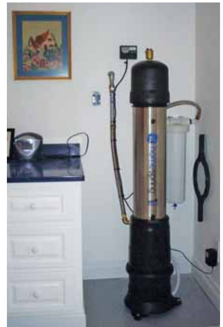
Harvested water flows through a sediment filter, an activated carbon prefilter and finally a backwashing ultrafilter.
