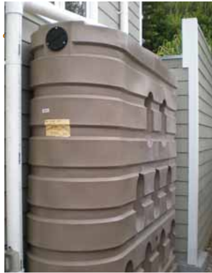
Rain barrels are a simple way to collect rainwater in residential applications. These barrels, located at California homes, come in a variety of shapes and sizes to fit homeowners' needs, and can be designed to blend in with a home's exterior.
