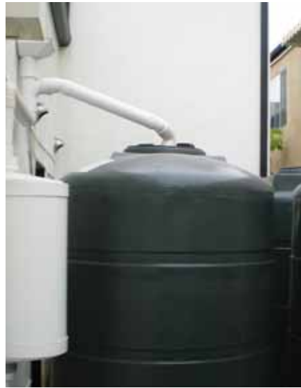
Rain barrels are a simple way to collect rainwater in residential applications. These barrels, located at California homes, come in a variety of shapes and sizes to fit homeowners' needs, and can be designed to blend in with a home's exterior.
