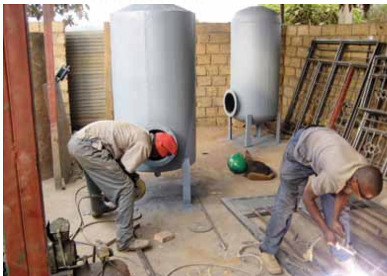
Left: Local welders put finishing touches on a filter body.
