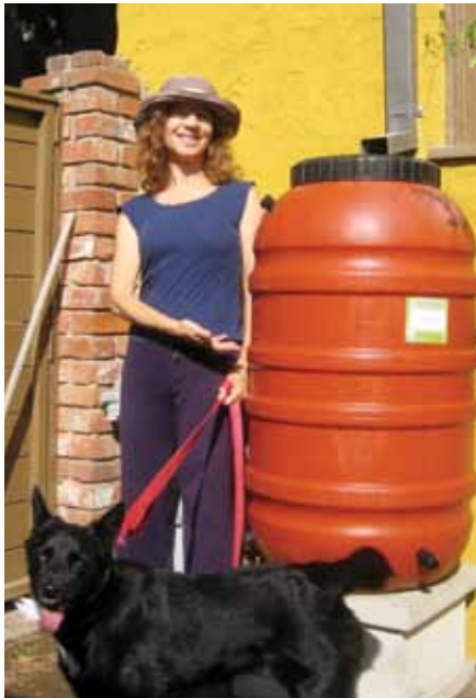
Kuntz, an early adopter of the rainwater harvesting program, with the rain barrel installed at her home
