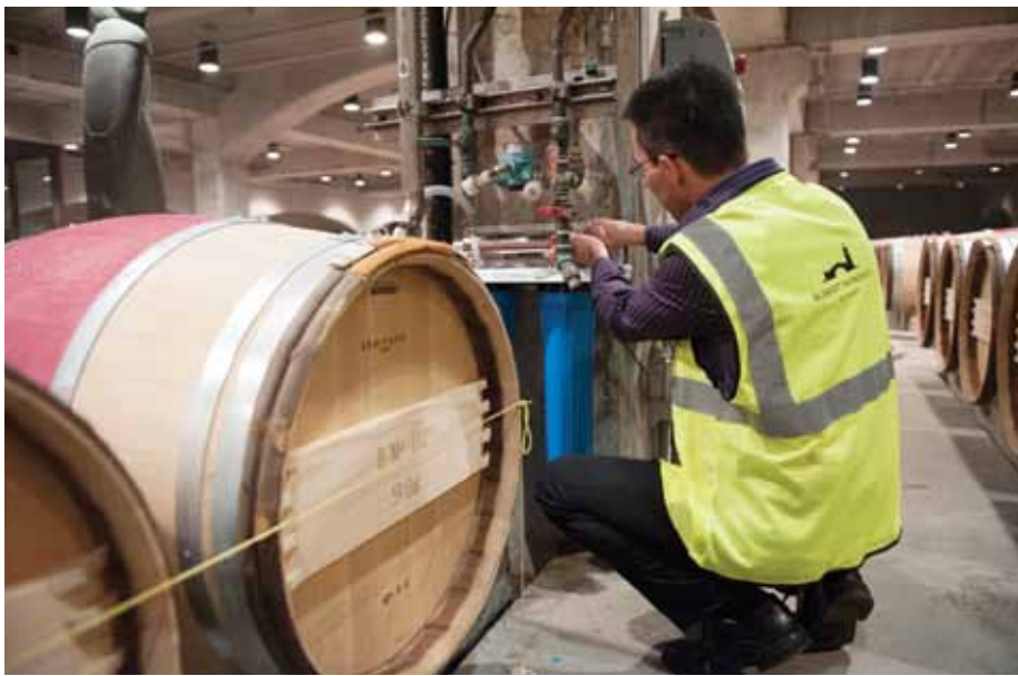
Jim Settle, founder of NuWater, installs the silica removal system, which helps prevent scaling and buildup in the barrel room's humidifiers.
