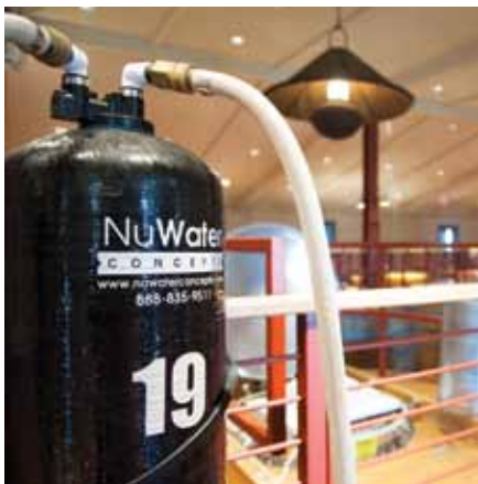
NuWater's system removes and destroys residual disinfectants from water to make it safe for barrel washing.
