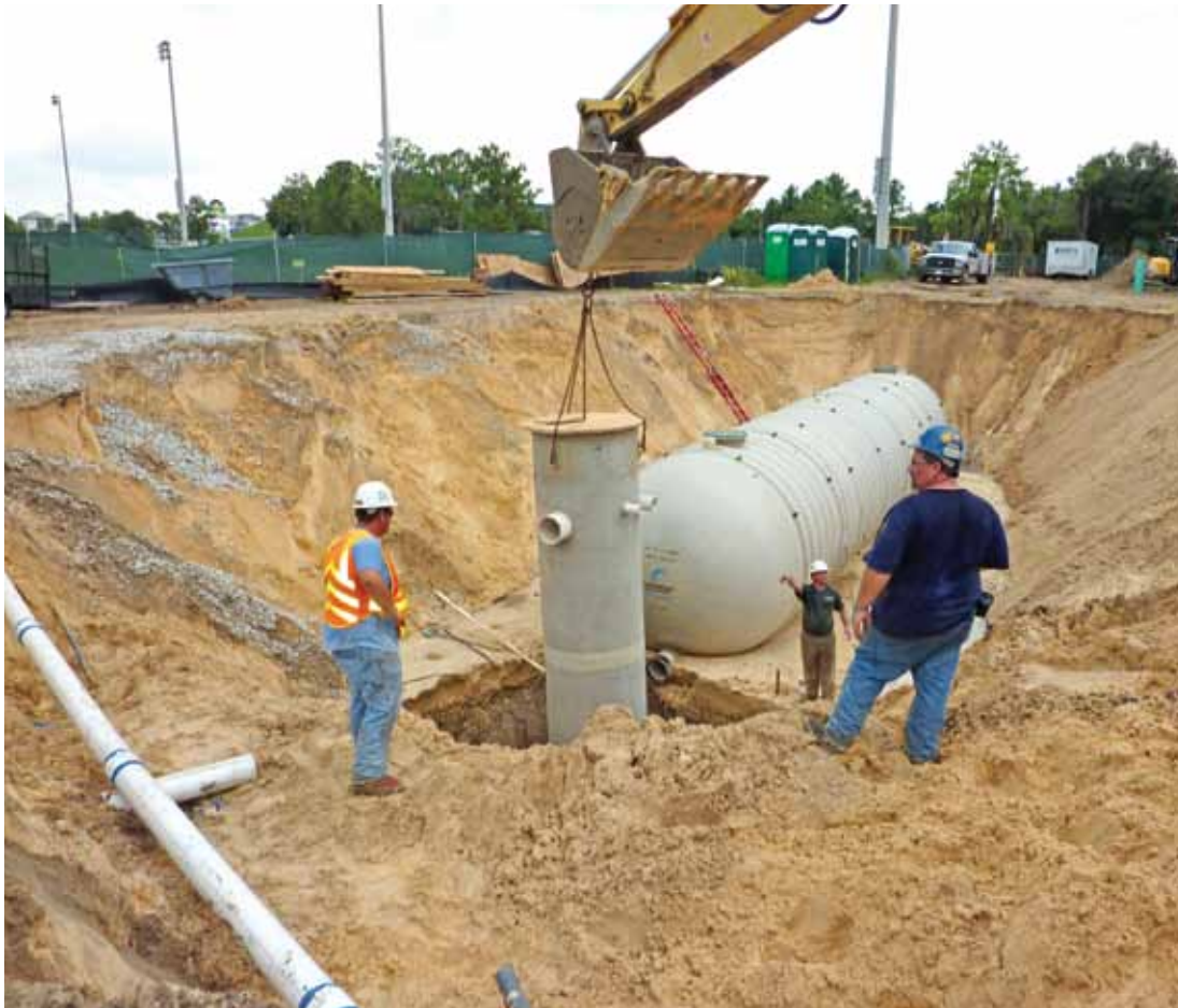
Top left: Placement of the 30,000-gal fiberglass tank required careful consideration, in an effort to avoid disturbing building foundations. Top right: The tank is connected to a backup system that switches over to the municipal water supply if tank levels get too low.
