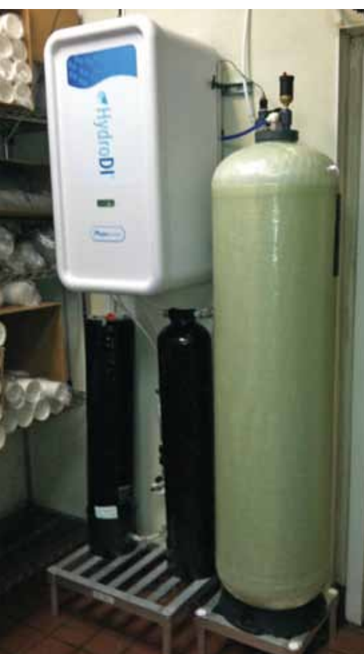
The water conditioning system allows a coffee shop to control the unwanted minerals and chemicals in its incoming water.
