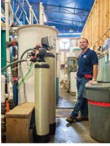
Owner Scott Cohen with the tanks containing the organic scavenger resin, which helps the facility cope with high levels of dissolved organics
