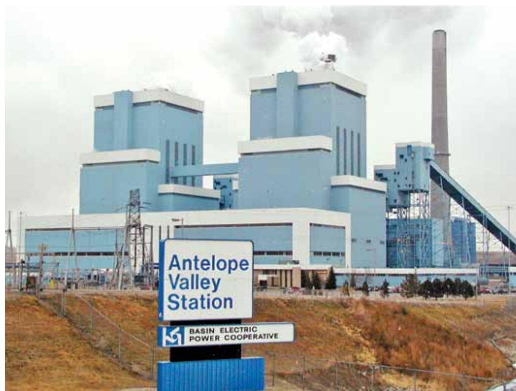
The Antelope Valley Station needed a cost-effective way to treat feedwater from its source, which is a reservoir of Missouri River water that contains concentrations of dissolved solids and silt.
