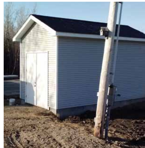
The arsenic removal system, housed in this building, serves 350 of the town's 1,500 residents.
