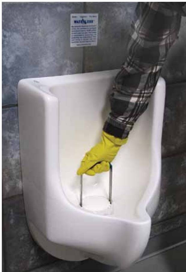
Proper maintenance is essential to ensuring that waterless urinals remain odor-free. Here, a staff member demonstrates how to remove a urinal trap.
