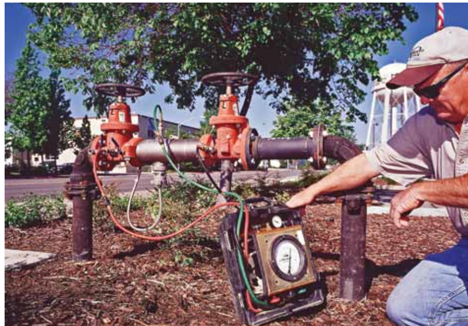
A technician measures the differential pressure across a backflow preventer's check valves.
