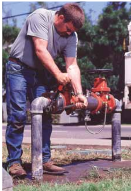
An installer completes a backflow assembly by tightening the flange.
