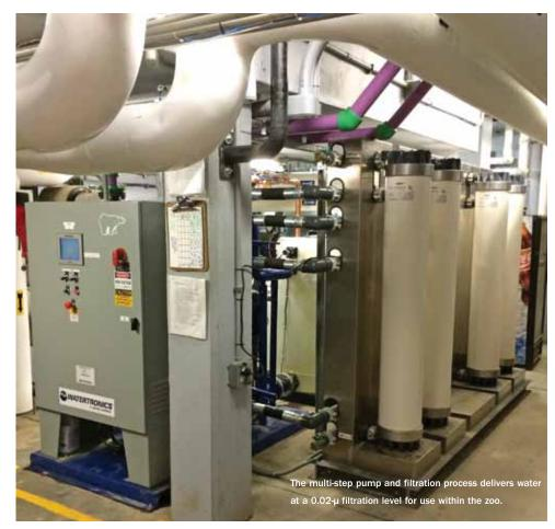
system, where it is filtered down to 0.02  $\mu-$  the virus level. For comparison, a human hair is 150  $\mu,$  and the naked eye cannot see anything smaller than 25  $\mu.$  UF systems like the one at the Cincinnati Zoo filter water to approximately 3,000 times smaller than a human hair.
