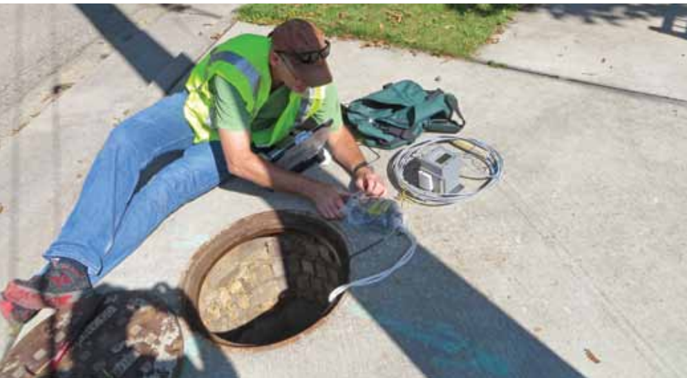
An MMSD employee troubleshoots a conductivity reader for manhole monitoring.
